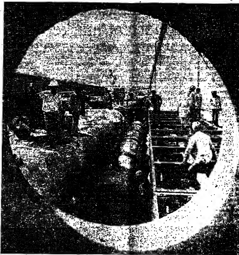
A drainage trench under construction in the floor of the main dock of the Dubai dry dock complex. The dock is being built by the Costain-Taylor Woodrow Joint Venture.
